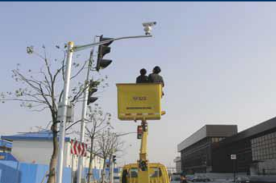
Construction in Pudong
