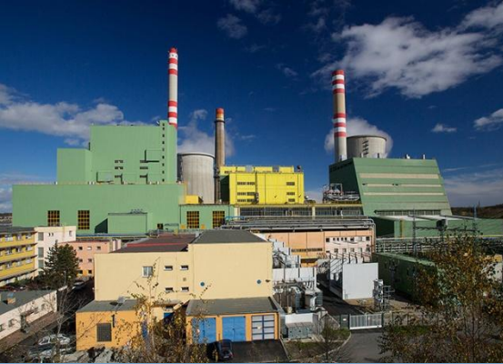
Heating Station in Kladno
